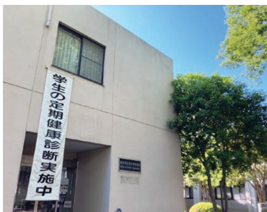
保健管理棟 Health administration building
