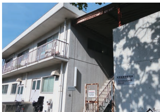
有害廃棄物管理棟 Waste management facility
